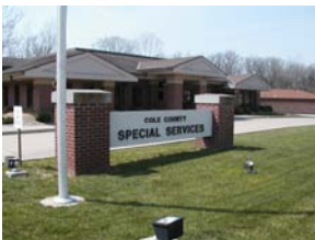
CCRSI MAIN OFFICE BUILDING.
